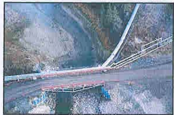
The lower bridge (above) after removal of the weir.
